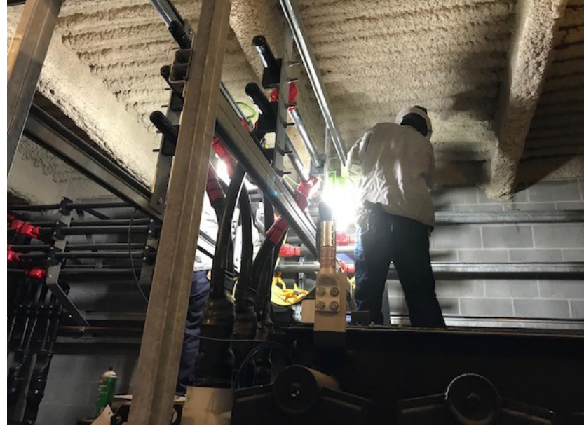
Figure 2: Journeyman replacing 480V secondary cables (Courtesy of www.impactaconsulting.com )
