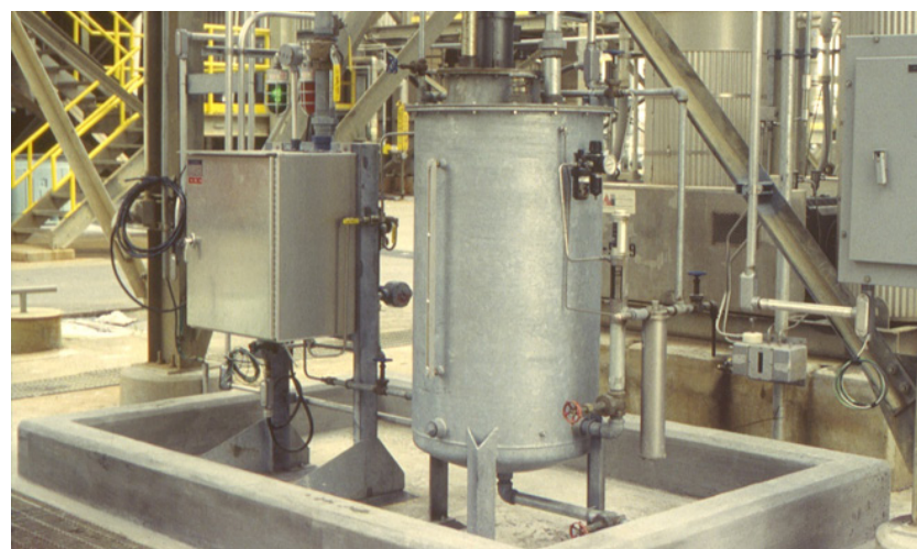
Figure 2: A medium-sized oil mist console is shown on the left; an oil return tank with its associated blower is positioned on the right
