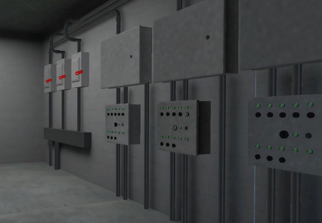
Figure 1: New 3-D simulation tools include PLC sensors that focus on teaching industrial PLC analog inputs, PLCs and associated devices
