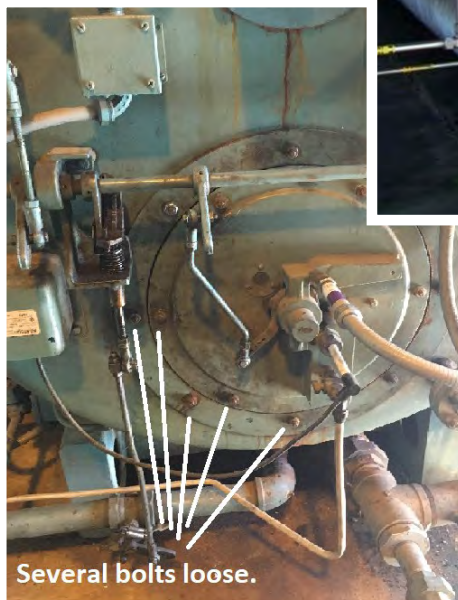
Figure 2: Horizontal flame box of a boiler
